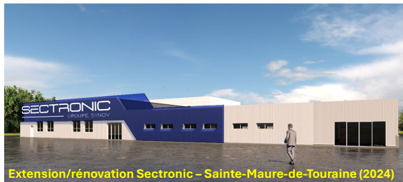
Extension/rénovation Sectronic – Sainte-Maure-de-Touraine (2024)
